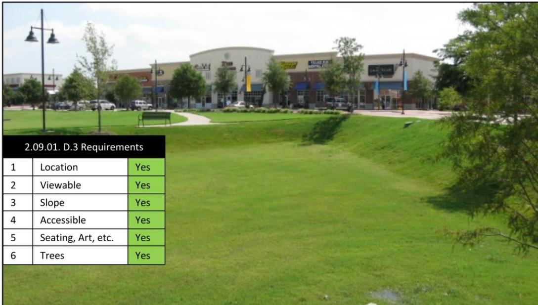
**Figure 4: Example of a Detention/Retention Pond Designed as an Amenity**
