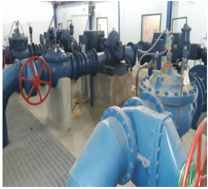
2 Water Pump Stations Repaired
