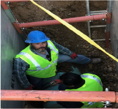
23 Water Main Repairs
