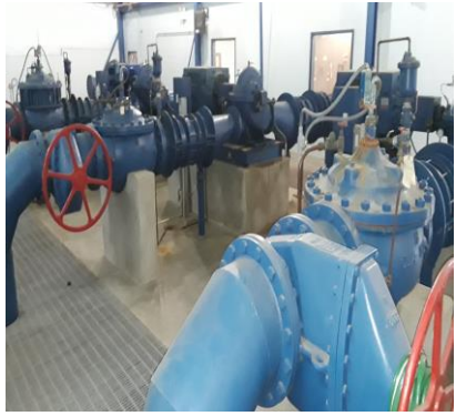
2 Water Pump Stations Repaired
