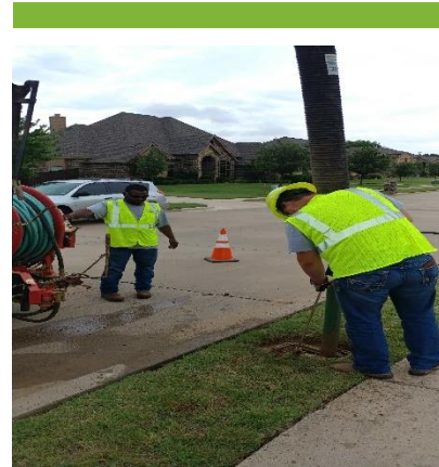
150 Meter Box Replaced & 75 Meter Sets
