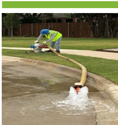
Flushed dead end lines 500 times
