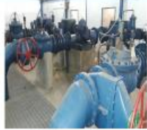
2 Water Pump Stations Repaired
