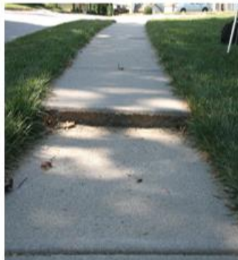
800 linear feet of sidewalk replaced
