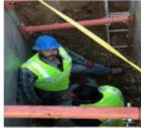
13 Water Main Repairs
