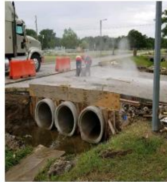
6,147 square yards of street reconstruction
