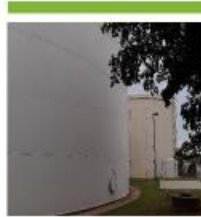
6 Water Storage Tanks Maintained
