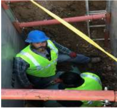
104 Water Line Repairs
