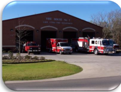
Fire House #2 2700 Shady Shores Road, Corinth
